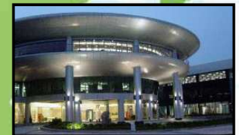
China Technology Center Shanghai, China
