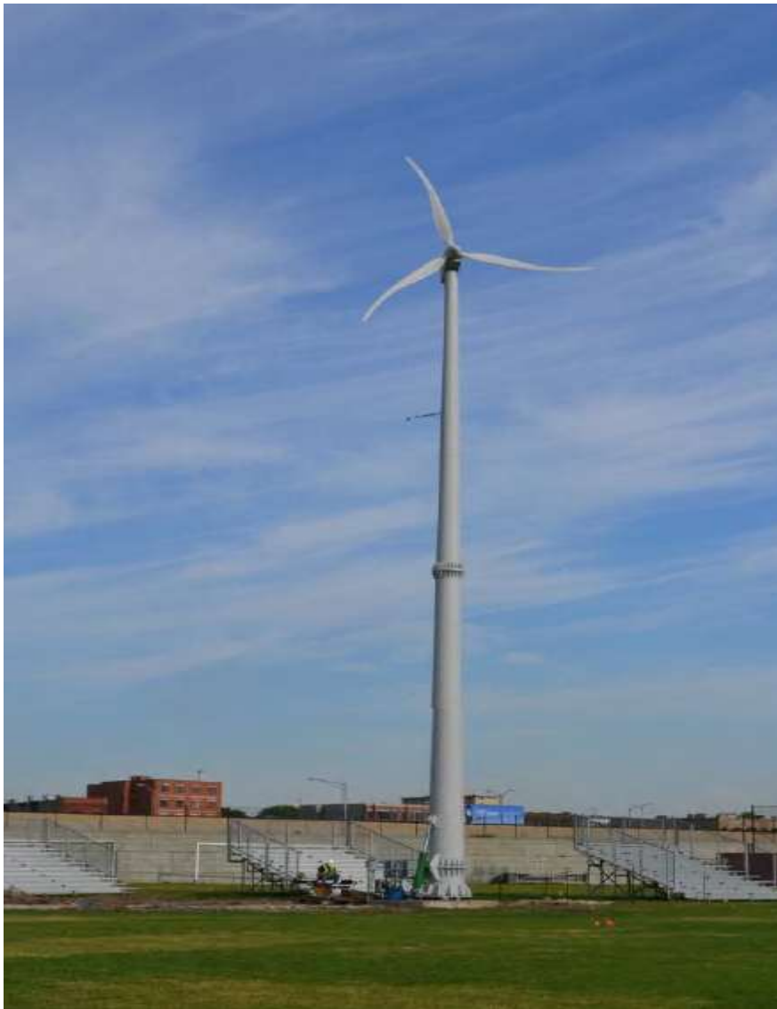
Figure 13: Viryd 8kW Unit Installed at the IIT Soccer Field
