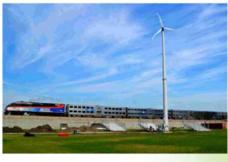
Figure 14: Installation Chronology for the Viryd 8kW Unit at the IIT Soccer Field
