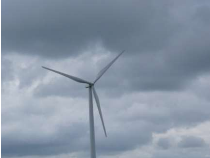
Figure 182: The GE 1.5 MW wind turbine located at the Invenergy wind farm in Grand Ridge, Illinois.
