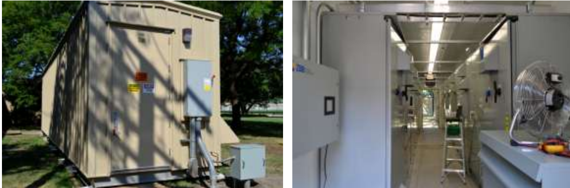
Figure 338: IIT Large-scale Battery Storage
