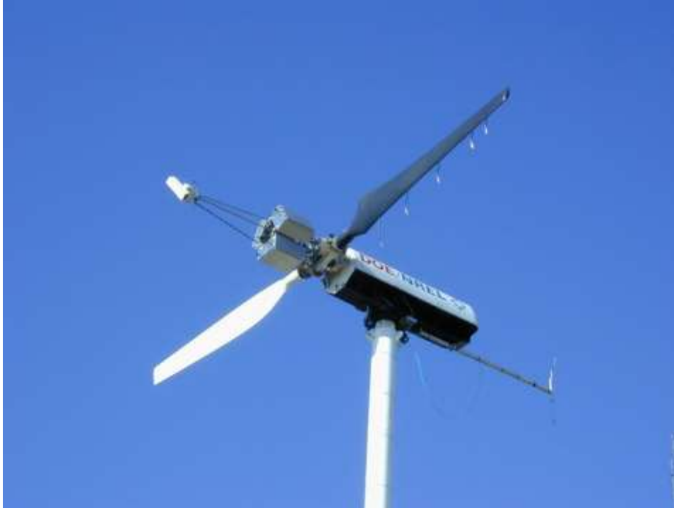
Figure 220: The NREL 10m research wind turbine
