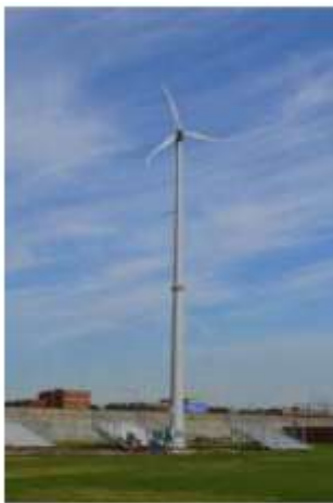
Turbine on Tower: 7/14
