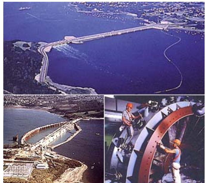
Figure 7. La Rance Tidal Power Station (Image courtesy of Popular Mechanics)
