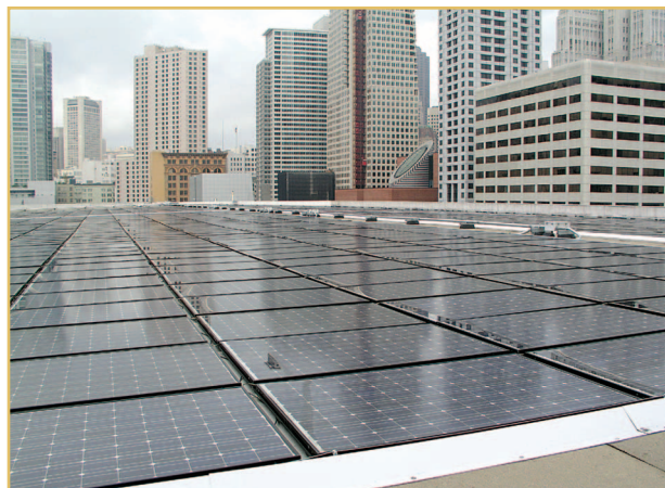
figure 7. View of San Francisco's Moscone Convention Center 675-kW PV installation (photo by Mike Kim, SFPUC).
