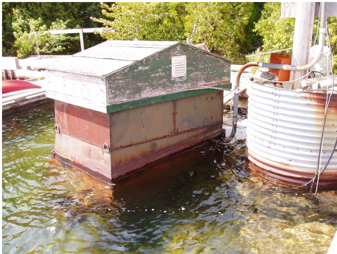
Fig. 3. Smaller of the two turbines at Laurentian Lodge
