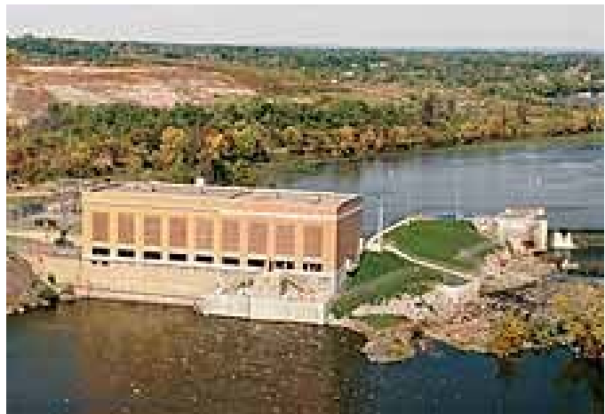
Fig. 6. Crescent small hydro plant on the Mohawk River
