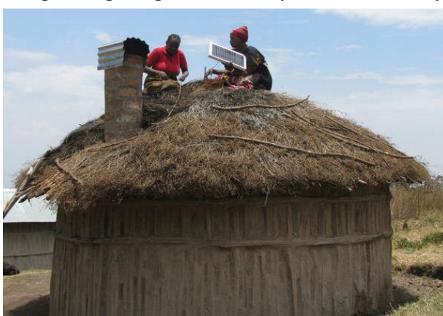
Figure 6: Helping locals install a prototype solar system on the roof of a house in Ghana (photos are taken by Dr. Shahidehpour)
