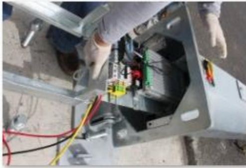
Carefully Insert the Cradle without Batteries Part Way in to the Bottom of the Tower
