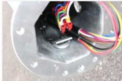
Detail using the Cable Connection Strain Relief Ties to Hook to the Tower
