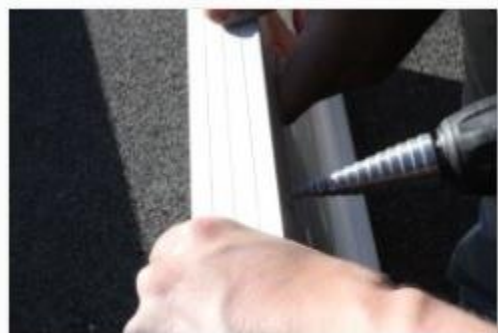
Mark Out and Drill Solar Panel Frame Carefully to Fit Bracketing
