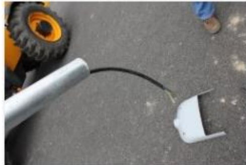
Pull Wire thru LED Light Armature
