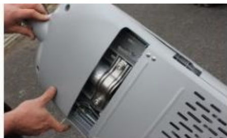
Replace Back Cover of LED Light
