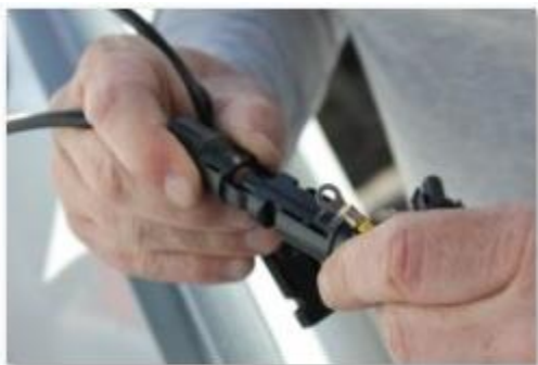
Connect Male and Female of Solar Connections
