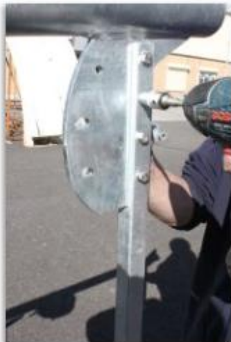
Tighten with Tool with Correct Torque Settings as per Table
