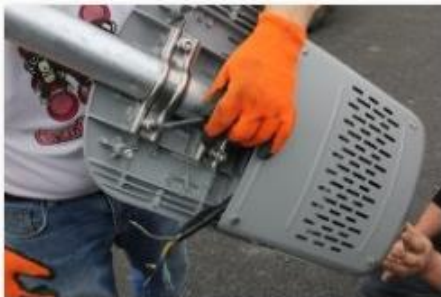
Align LED so it will Face Down when Tower is Erected and Tighten with Allen Key
