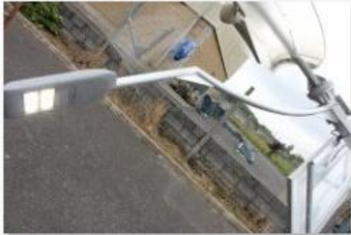
Test All Connection Before Raising the RPU System
