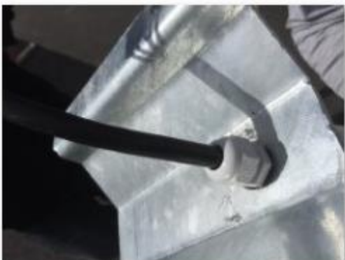
Screw Gland into Hole to Protect LED Wire
