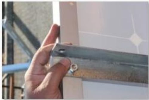
Fix Bracketing to Solar Panel as per Drawings
