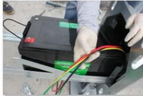
Fully Insert First Battery and Slide Cradle in another Third Way
