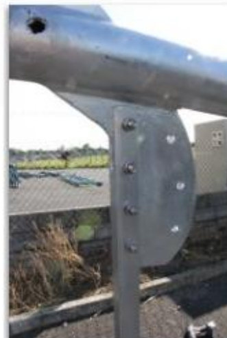
Tail Fin Secured(Being Replaced with Lock Nuts)
