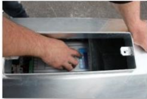
Check Charge Controller Settings and Operational Status
