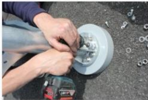
Connect Bearing Using the Bolts Provided
