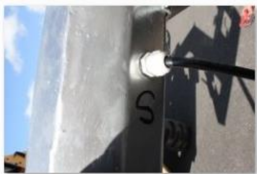
Connect Gland To Solar Panel Connection Loom and Fix it to Tower
