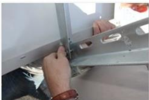
Attach Solar Bracketing to Solar Armature as Per Drawing
