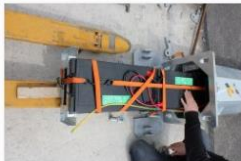
Use Extra Straps if Necessary to Secure Batteries in Place (Straps To be Replaced with Bracket).
