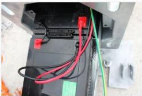
Battery Cables Connected
