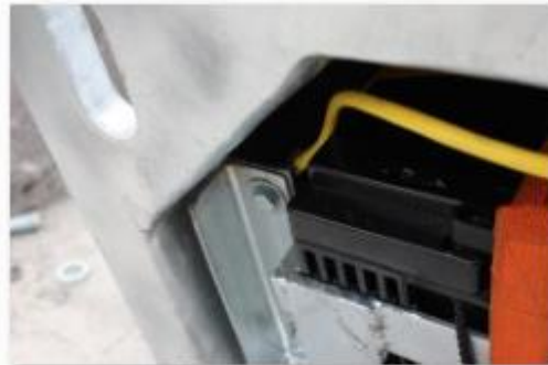
Fix Earthing Wire to Earthing Point at the Base of the Tower
