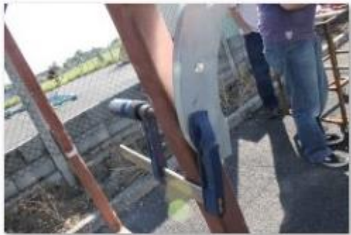
Clamp Stiffner Bracket To Prevent Generator Pole from Rotating
