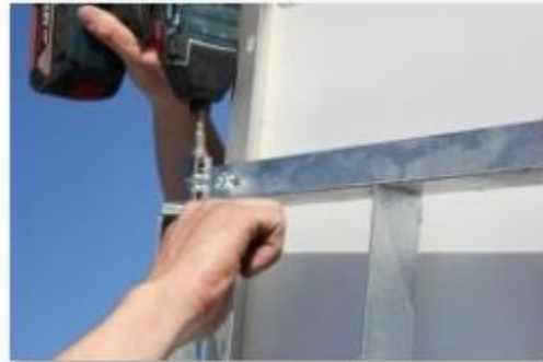
Tighten using Tool with Correct Torque Setting
