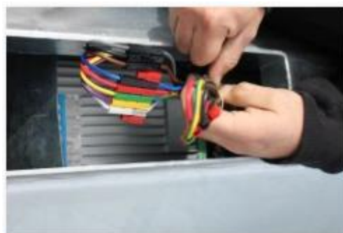
Connect Cables from the Cradle to the Wiring Looms in the Tower
