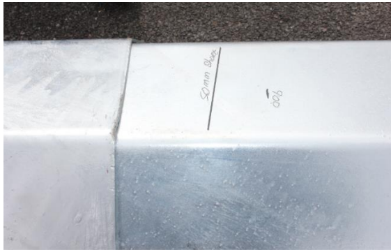
Slip Joint on the Tower Showing 900mm Stop Dimension
