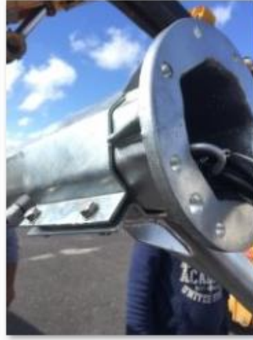
Offer Up LED Armature Clamping Bracket and Tighten Equally All 4 Nuts
