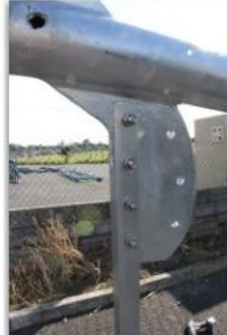
Tail Fin Secured(Being Replaced with Lock Nuts)
