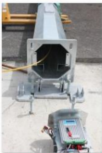
Feed 'Pull Wire' thru Tower
