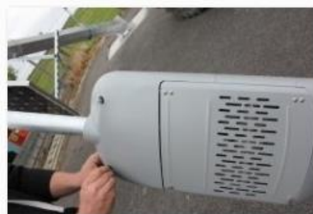
Securely Screw Fixings to Secure Back Cover with Hand and Tighten with Flat Head Screwdriver
