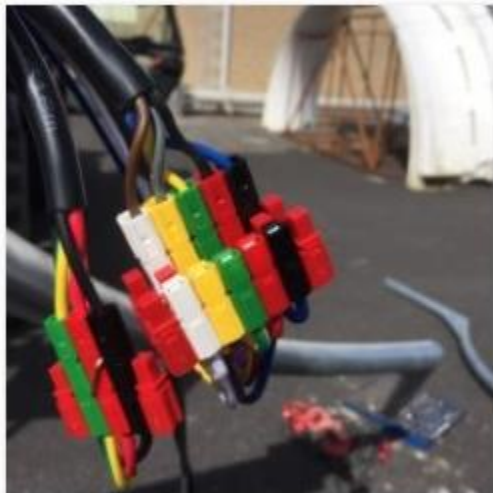
Ensure Looms are Connected before Connecting Poles
