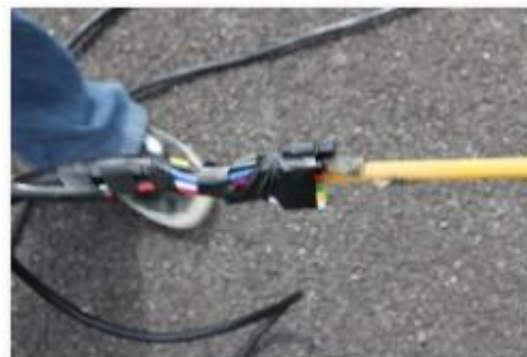
Connect Securely and Tape Cables to be Pulled thru Tower
