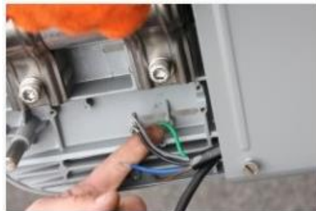
Connect Earth to LED Grounding Point
