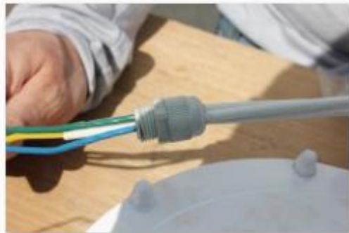
Put Cable Gland on Wire from Generator and use 'Pull Wire' to pull it thru Pole to Bearing
