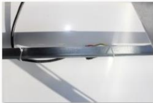
Fix Earthwire to Solar Panel Frame and Use Cable Ties to Tidy Away Cabeling at the Back of Solar Panel
