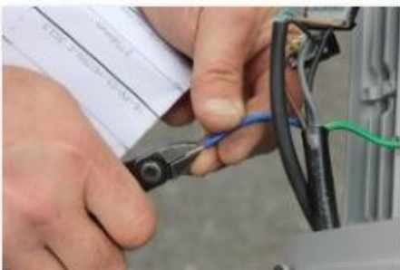
Prep LED Light Cables for Connection via Terminal Block
