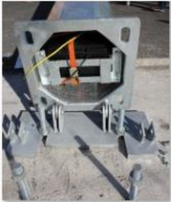
Ensure that the Cradle is Bolted into Position
