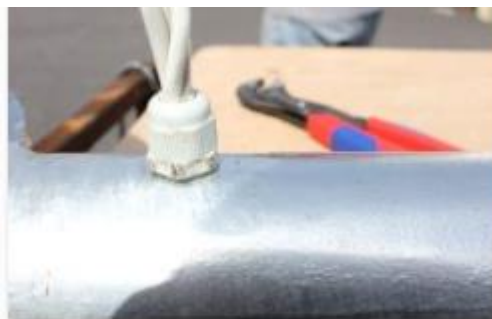
Generator Cable Gland Connected
