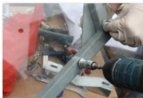
Tighten Fixings with Tool with Suitable Torque Setting Available
