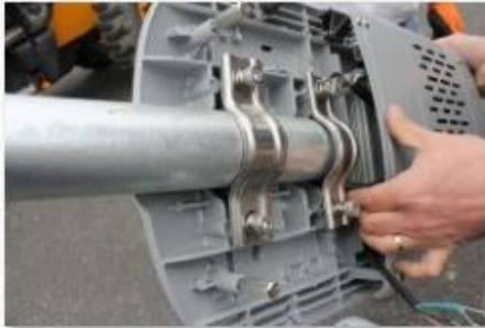
Unscrew and Remove Back Cover of Light, Loosen Fixings and Slide LED Light on to Armature
