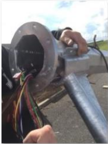
Offer up the LED Armature and LED Wire to the Tower and Connections to Loom
