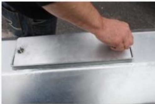
Replace Access Panel Cover Plate and Hand Tighten Fixings
