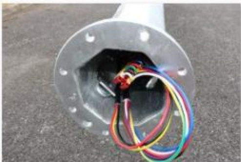
Use the Cable Connection Strain Relief Ties to Hook to the Tower
