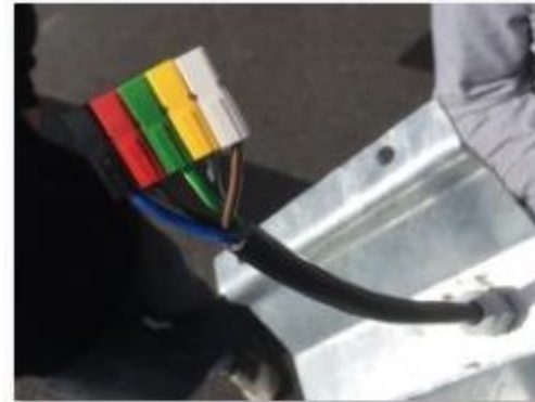
LED Armature Wired
