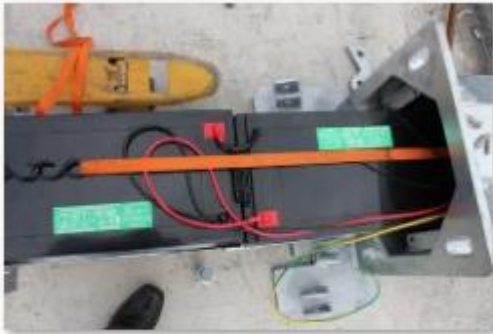
Secure Batteries in Place with Strap (To be Replaced with Bracket)
