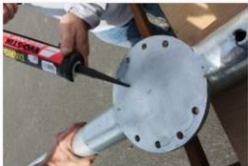
Prep Surface of Generator & Mounting Plate with Silicon, Then Place Anti-Resonance Rubber
