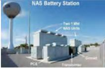
Three 2MW NaS Battery installations in AEP distribution system, 2008
