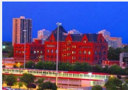
The Illinois Institute of Technology in Chicago, home to a unique nanogrid in a microgrid
