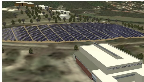
Figure 9. The UVI St. Thomas Campus 2,099-kW dc solar array.
