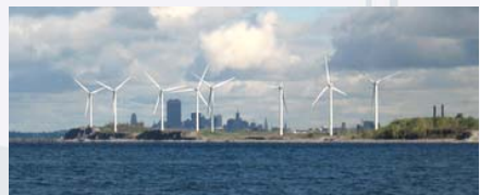
Steel Winds Project on the Buffalo Waterfront
