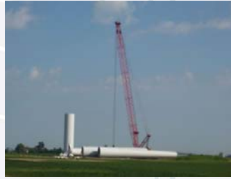
Construction of Port Alma Wind Farm
