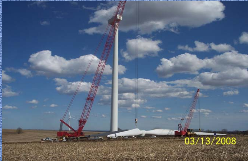
The assembly is ready to be lifted.
