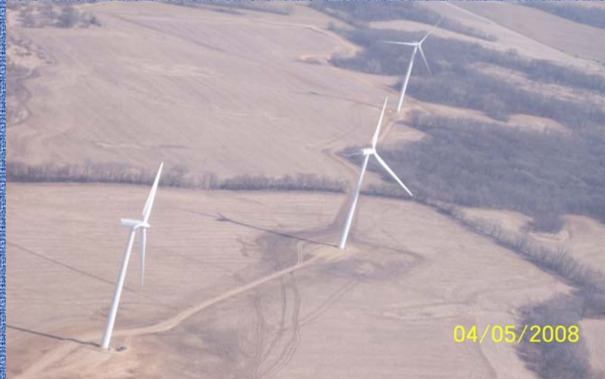
Aerial view of the completed towers.
