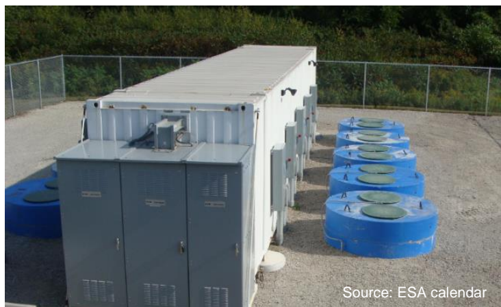
Beacon Tyngsboro, Flywheel, 1MW, 250 kWh
