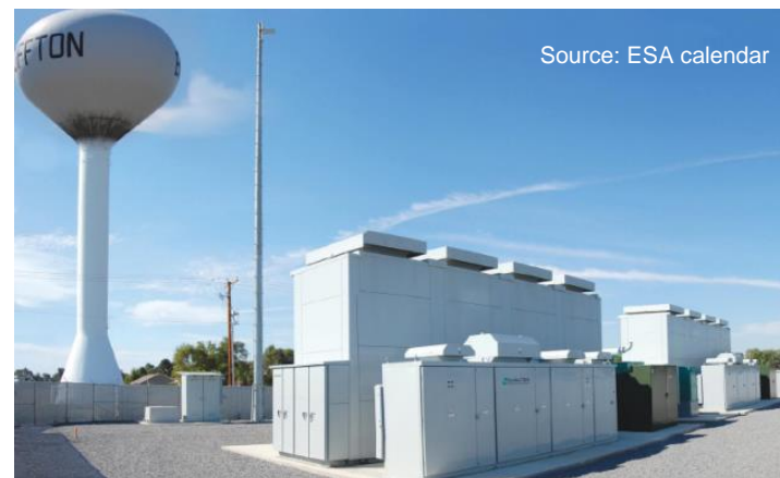
AEP Bluffton, NaS, 2MW, 14 MWh
